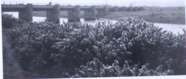
The Annan River viaduct or bridge after Lichminster.
