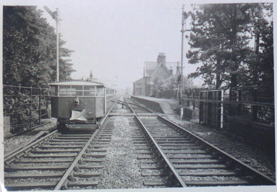
14 maintenance trolley at the North end of Ingleton Station (MID)
