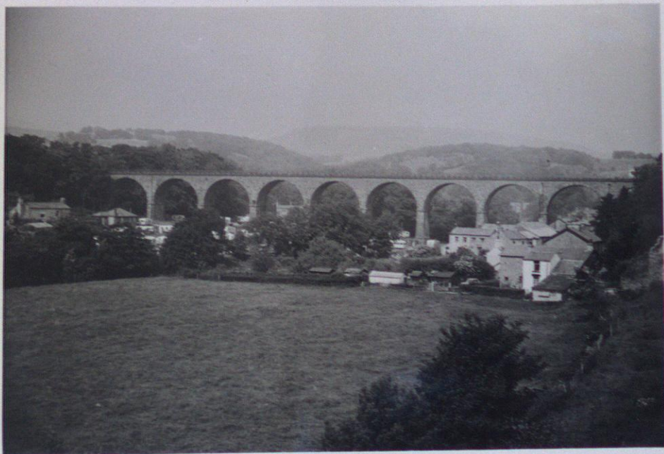
Ingleton Viaduct - I took this before I got to the station!
