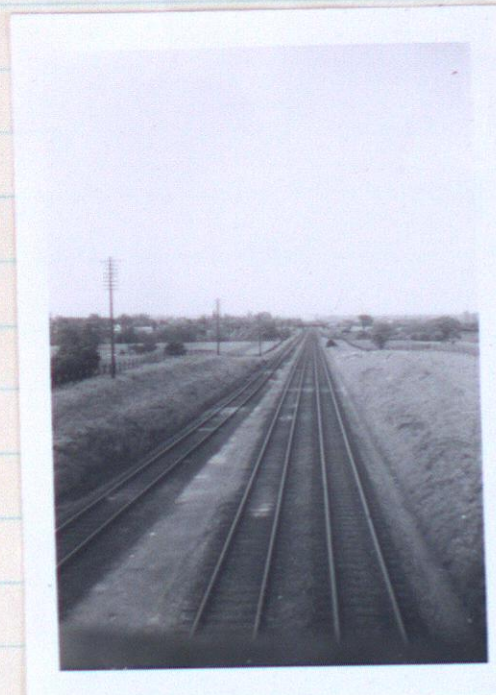
A strip of G. W. R. track illustrating the gap left by the broad gauge. (No!) Broad Gauge only reached Wolverhampton.
